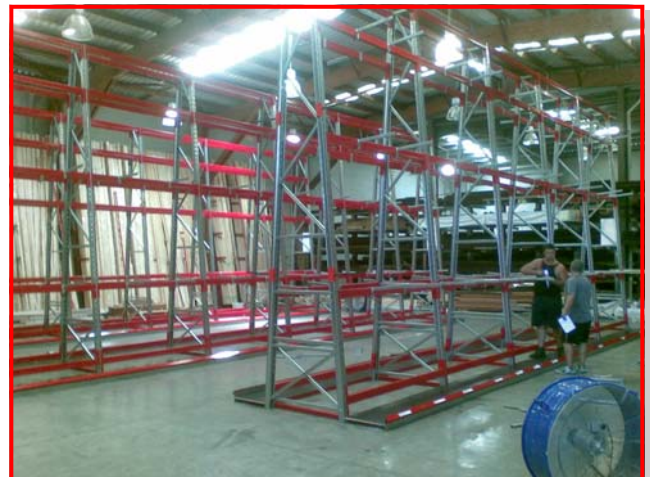
The engineered and certified Macrack system installed to replace the timber A-Frame racking.
