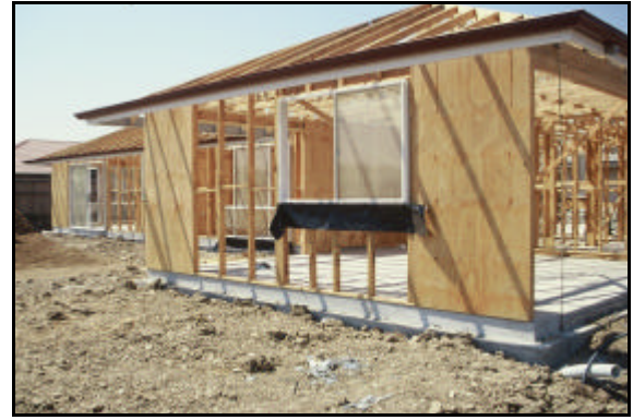
About 90 per cent of Australian homes are built using timber framing.
