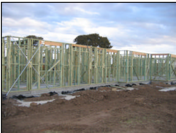
Blue Pine framing utilising an envelope treatment with environmentally friendly pyrethroids is backed by a 25 year guarantee and effective against termite and European house borer attack.
